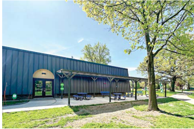
Opposite page: Top 1 & 2: The Fieldhouse+ project displays a double-facade system with insulated metal panels (IMPs) and perforated panels. Renderings courtesy of RODE Architects
