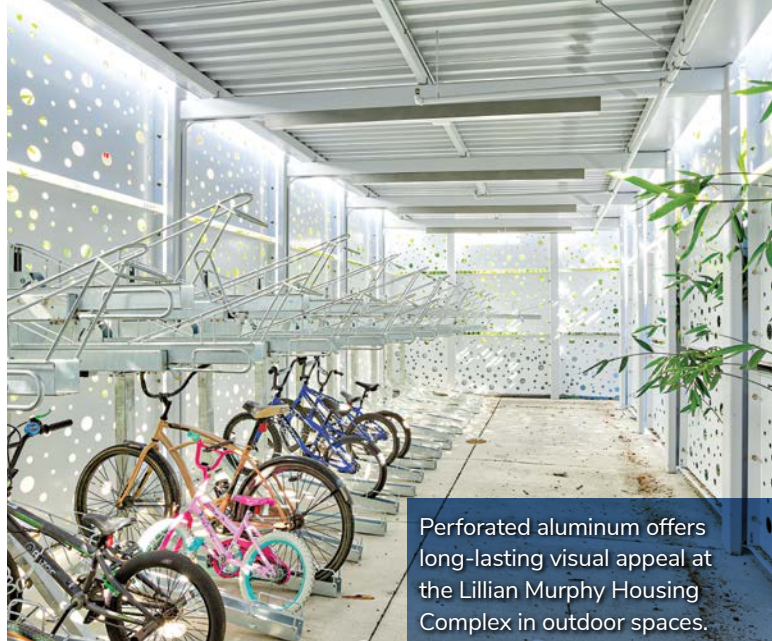
Safety, airflow, and daylight permeability are all supported by the perforated metal guardrails on the Lillian Murphy Housing complex exterior corridors and balconies.
