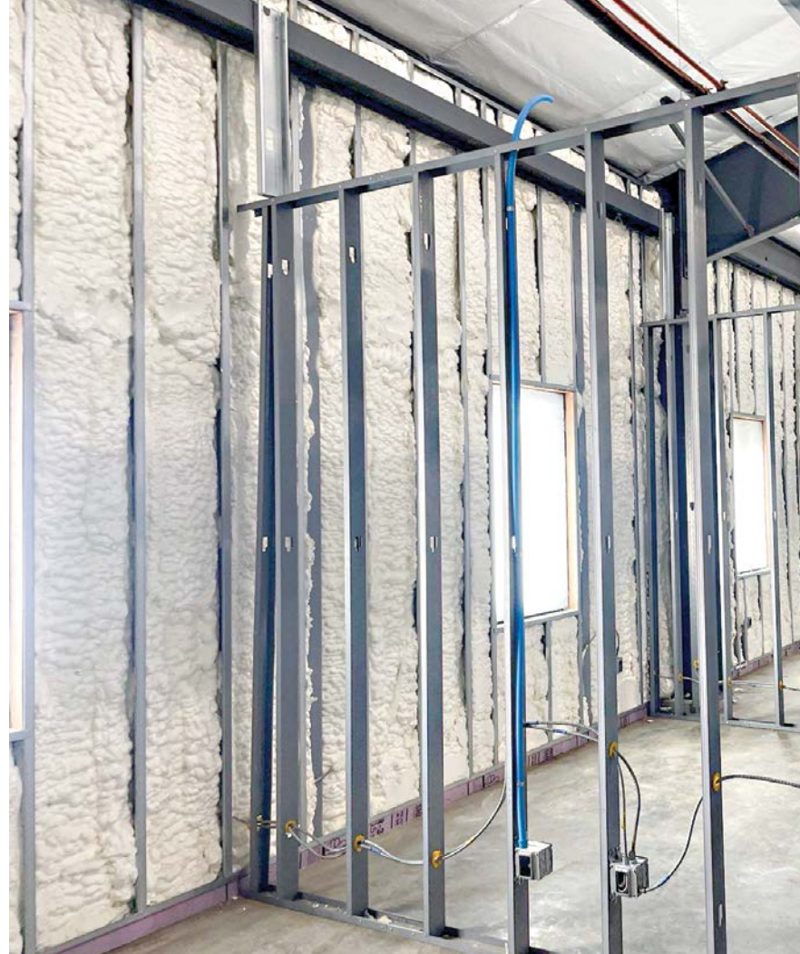
Exposed insulation is increasingly used as a visual design feature, with various clean and sleek options.
