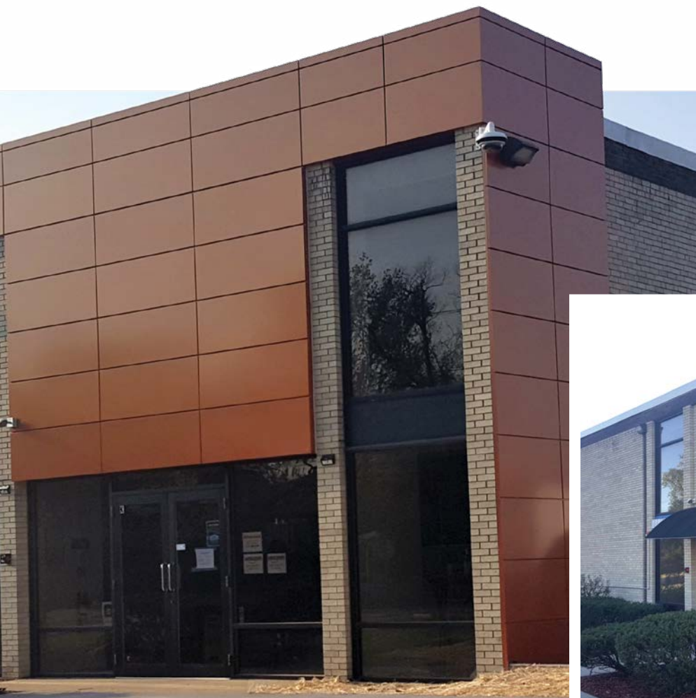
The building owner at 1951 Landmeier in Elk Grove, Ill., took advantage of the village's facelift incentives to improve the appearance of the building with a lightweight aluminum rainscreen. Photos courtesy Sheet Metal Supply
