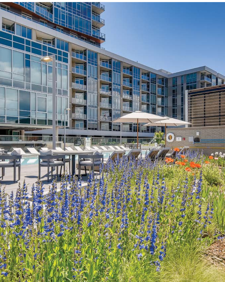
Photos courtesy Nava Real Estate Development
