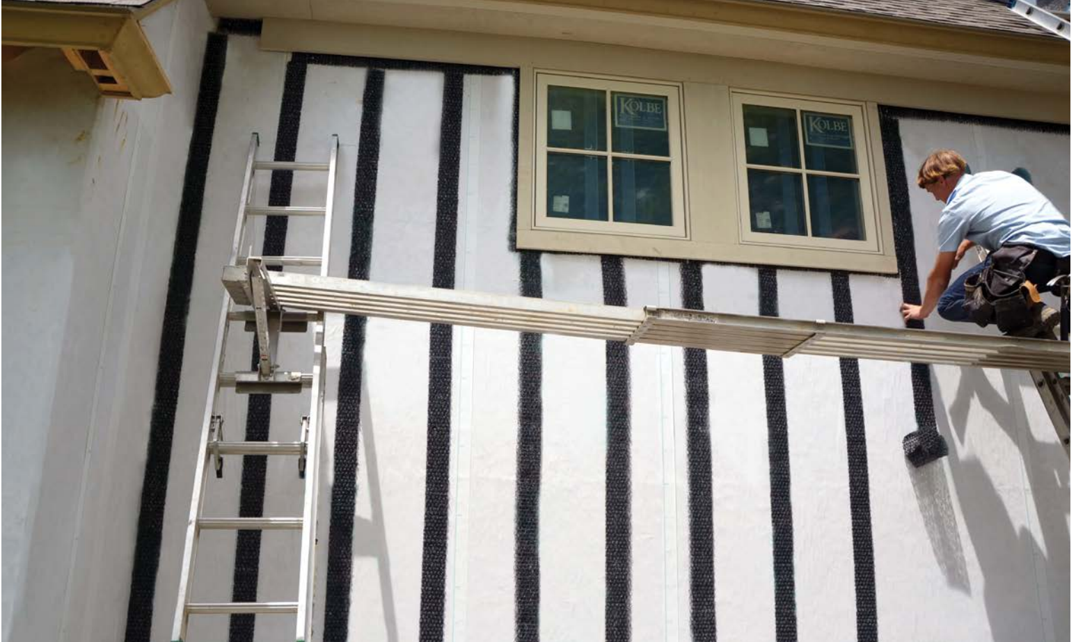
The installation of a rainscreen system on a residential facade.
