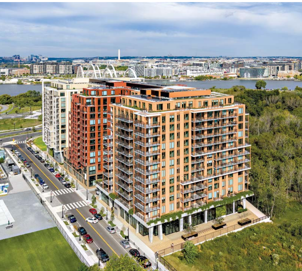
The Bridge District Phase 1 in Washington, D.C., uses 0.125 in. (3.175 mm) aluminum plate and aluminum composite material in a highly customized mixed-use residential facade.
